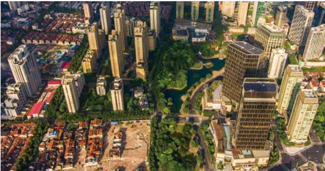
Overview of Shanghai Taipingqiao
