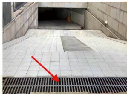
Trenches for entrances to the basement
